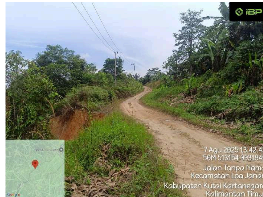
Before the construction of the temporary diversion road due to the landslide in RT 13
