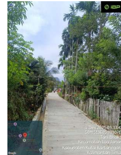
After the road concreting programme in Tani Bhakti Village was completed
