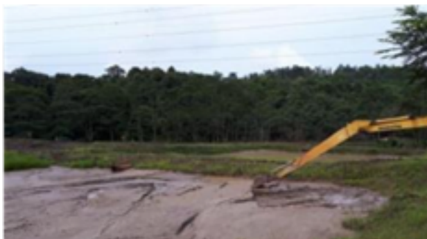
Kegiatan pengerukan sedimen di Settling pond/ Sediment dredging activities at Settling pond
